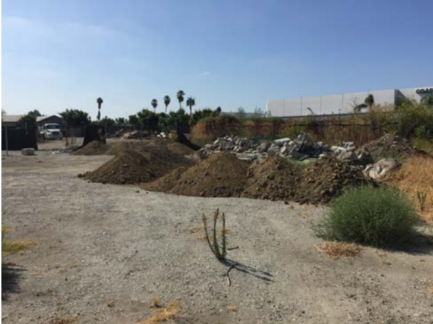
Photograph 13. View of the soil and concrete debris piles on the central area of the subject property, facing south.
